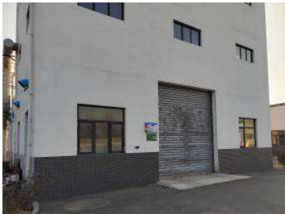
污泥脱水机房密闭
