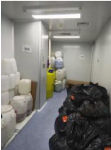
4 幢危险废物暂存间地面防渗及托盘
