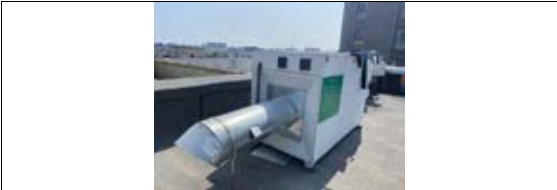
DA001 废气排放口现状
